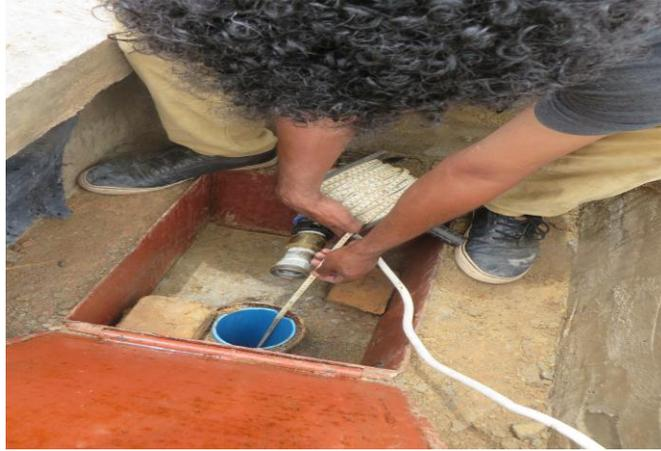
Install the pulley/tripod at the head of the borehole, in front of borehole diagnostic tool car.
