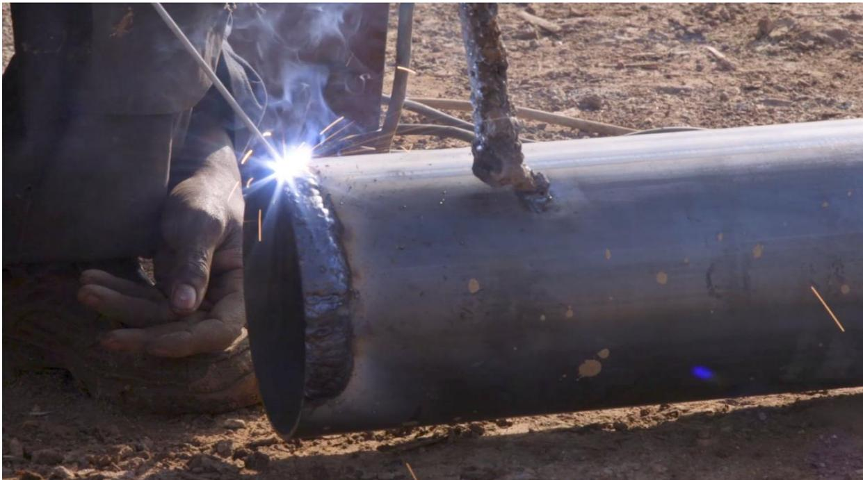
**Figure 10: Reinforcing the bottom of the steel casing**
