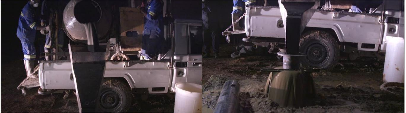
Figure 18: Pouring of grout inside the steel casing
