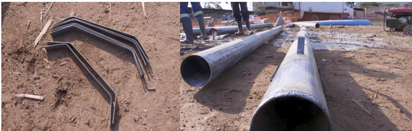
**Figure 11: Centralizers to keep steel casing straight down the hole**
