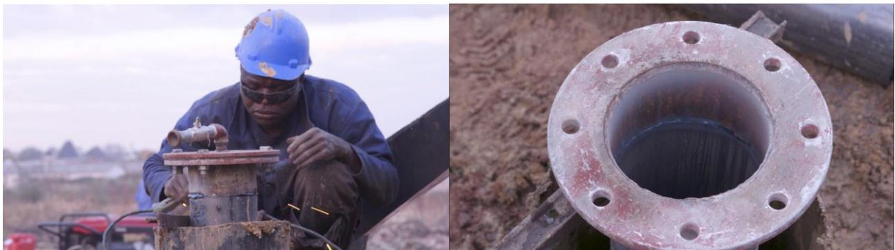
**Figure 15: Welding of the flange on the top of the steel casing**
