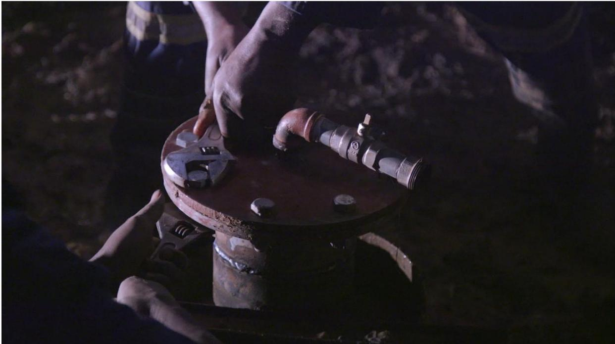
**Figure 20: Fitting back the upper part of the flange with a gasket and valve**
