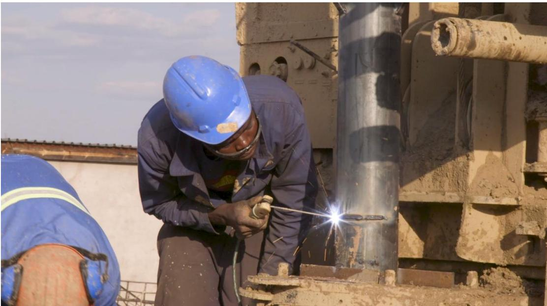
**Figure 13: Welding of two steel casings together while lowering down the borehole**
