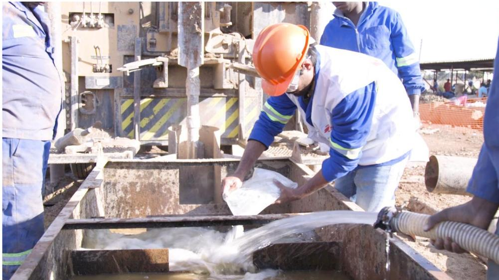
**Figure 7: Drilling mud being sprinkled on the water jet for homogenous mixing**
