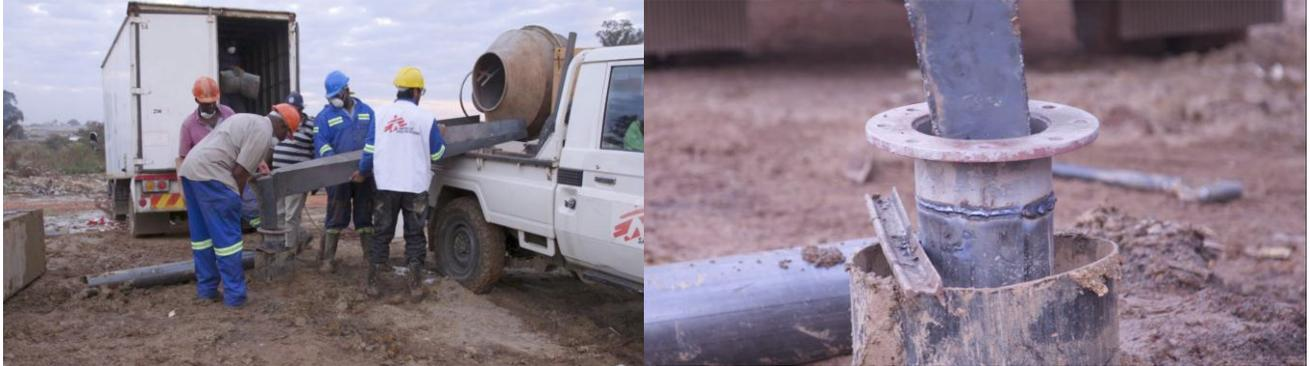
Figure 17: Adjustment of concrete mixer and funnel above the borehole
