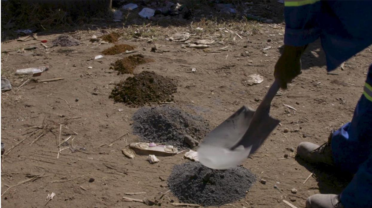
**Figure 6: Borehole cuttings during drilling of the pilot hole (DTH hammer drilling technique)**
