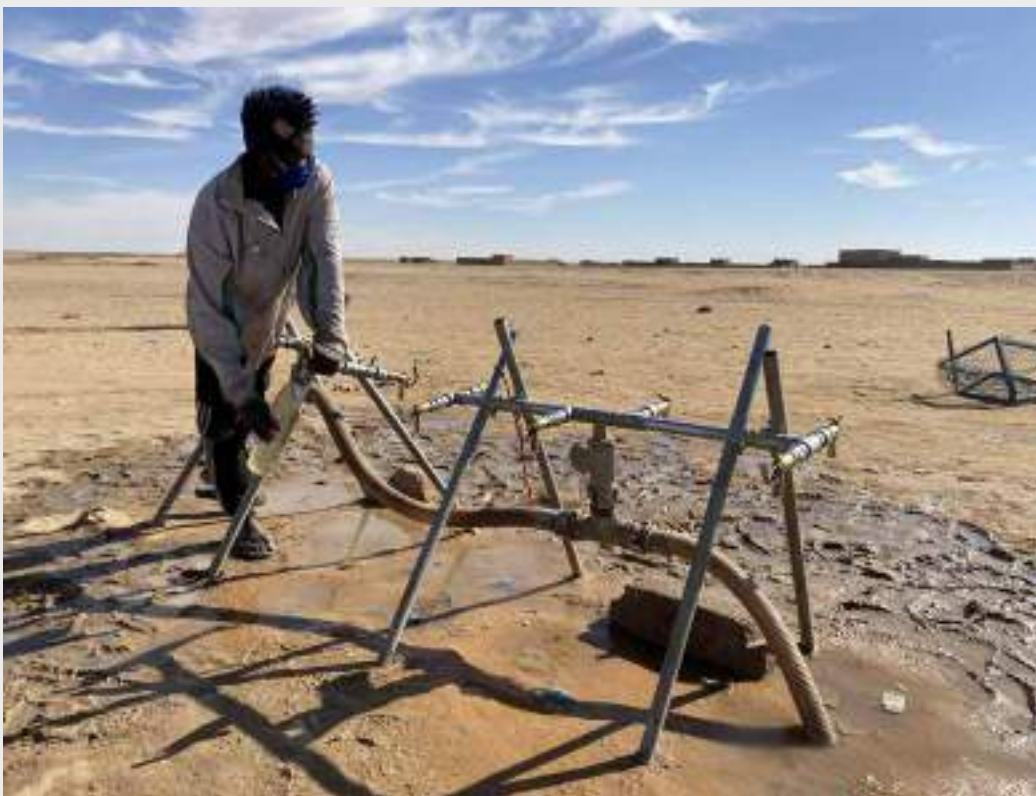
A young man fills a water bottle at a pump installed by MSF in Assamaka, Niger, November 2020. © Mariama Diallo/MSF
