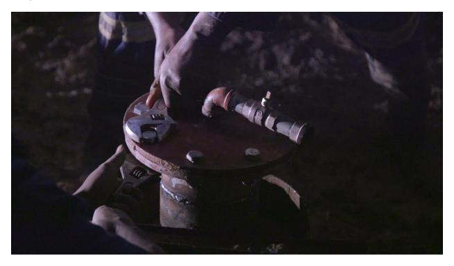
Figure 20: Fitting back the upper part of the flange with a gasket and valve
