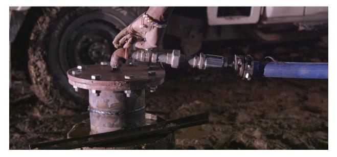
Figure 22: Closing of flange valve to maintain the pressure
