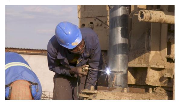
Figure 13: Welding of two steel casings together while lowering down the borehole
