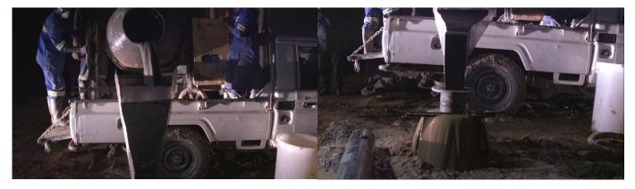
Figure 18: Pouring of grout inside the steel casing
