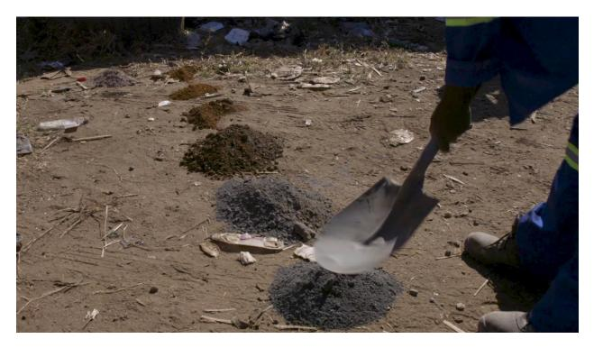
Figure 6: Borehole cuttings during drilling of the pilot hole (DTH hammer drilling technique)
