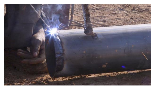
Figure 10: Reinforcing the bottom of the steel casing
