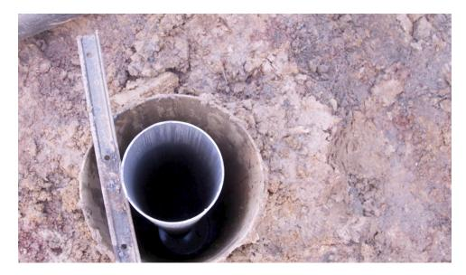
Figure 14: Steel casing assembly hanging in the borehole with a support of a metal bar welded at the top
