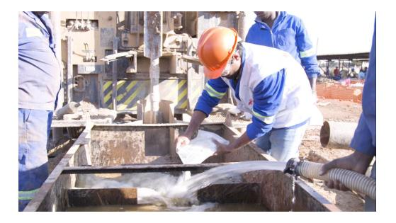
Figure 7: Drilling mud being sprinkled on the water jet for homogenous mixing
