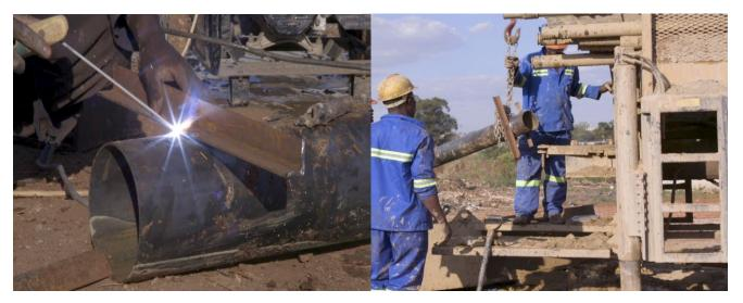
Figure 12: Lowering the steel casing into the borehole
