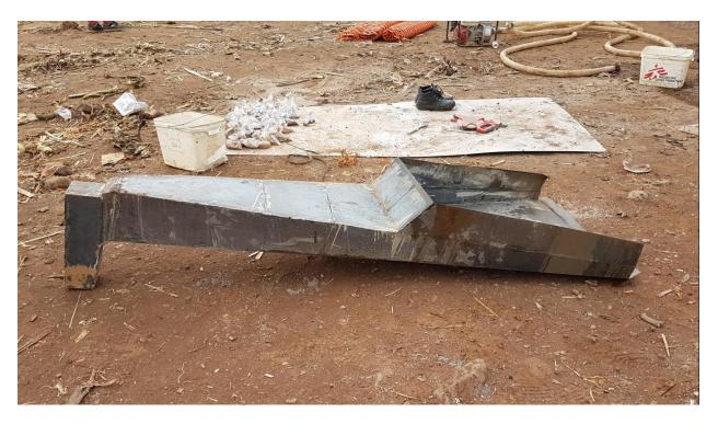
Figure 16: Custom made funnel to pour the concrete inside the borehole
