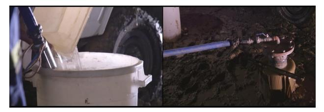
Figure 21: Water being injected inside the steel casing
