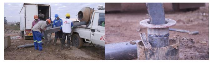
Figure 17: Adjustment of concrete mixer and funnel above the borehole
