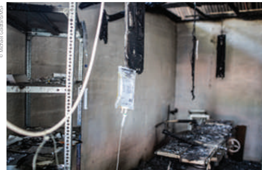
MSF's hospital in Leer, South Sudan, was looted, burned and destroyed, along with most of Leer town in early February, 2014. Hundreds of thousands of people were cut off from critical, lifesaving medical care. Opened by MSF 25 years ago, it was the only secondary healthcare facility in Unity State.
