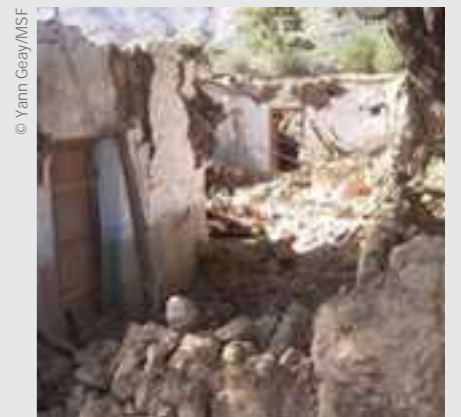
Building devastated by the earthquake in Pakistan
