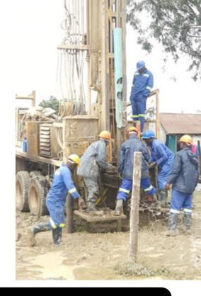
Through its WASH program, MSF has rehabilitated 70 existing boreholes providing safe and sufficient water to communities and institutions like churches, clinics and schools across Harare since 2015. These boreholes were rehabilitated using a unique borehole diagnostic tool kit, mounted in a self-contained vehicle.
