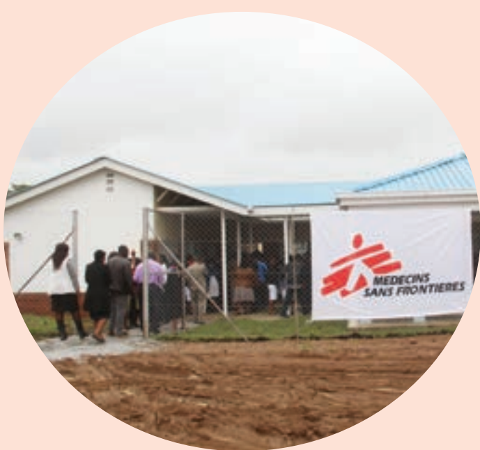
Newly constructed out-patients department (OPD) at the Harare Central Hospital Mental health Unit
